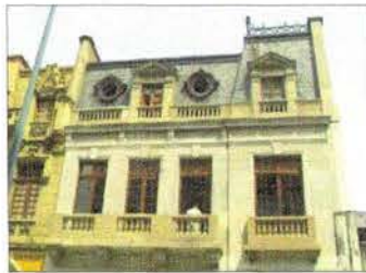
Vista fachada principal
