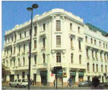
Vista fachada principal
