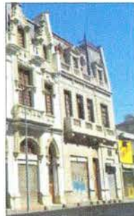
Vista fachada principal
