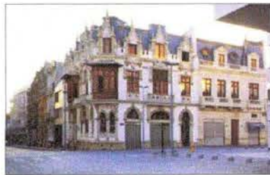
Vista fachada principal
